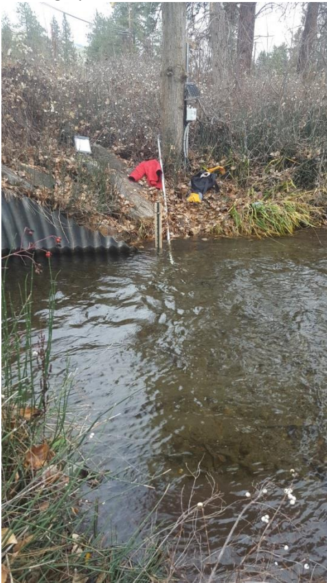
Looking right bank to left bank
