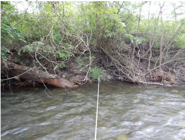
Looking right bank to left bank
