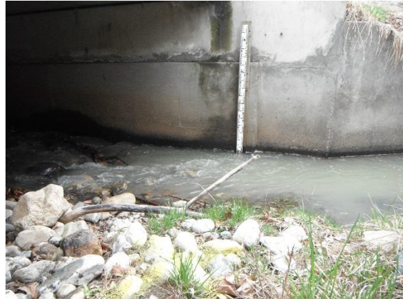
Staff gauge at Maple Street bridge
