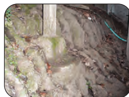
Visible erosion under a deck is common.
