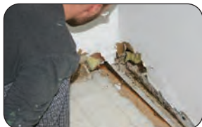
Repairing mold and water damage
