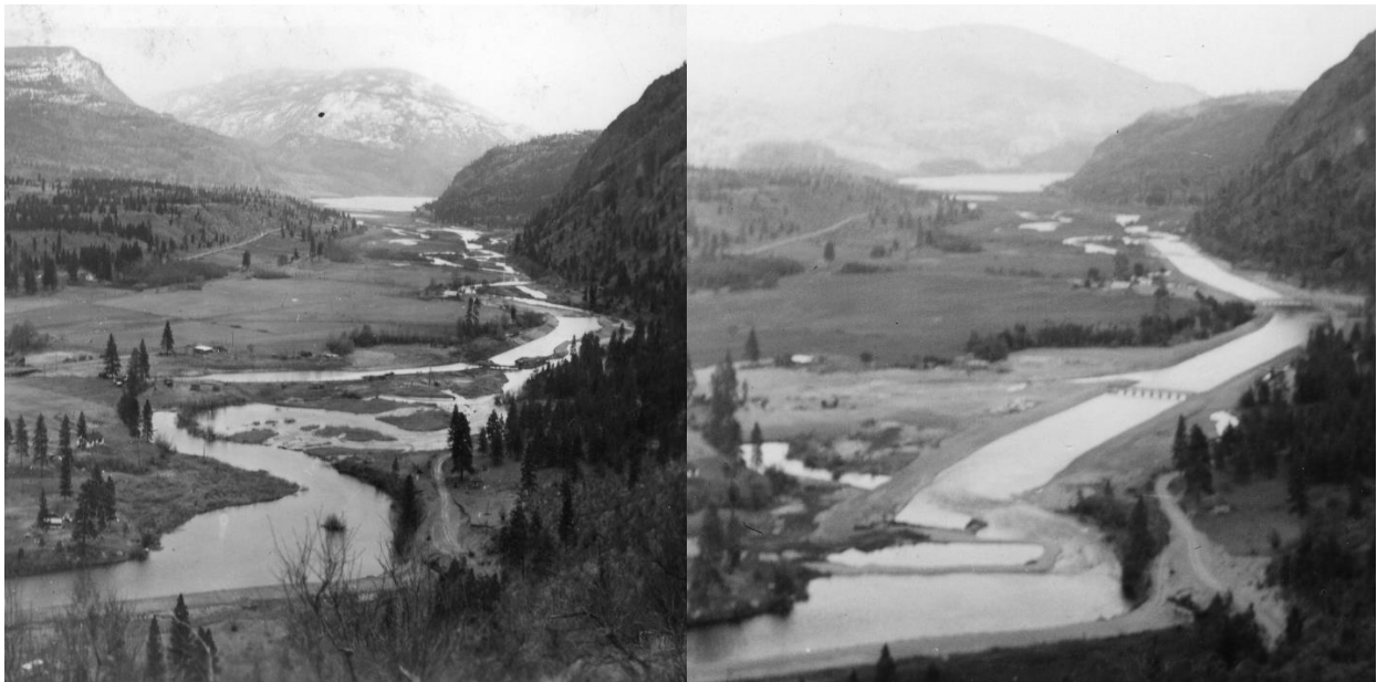
Figure 8. Historic photo comparison of Okanagan Falls (left) looking south in 1953 and in 1954 (right) after channelization (Courtesy of Penticton Museum).
